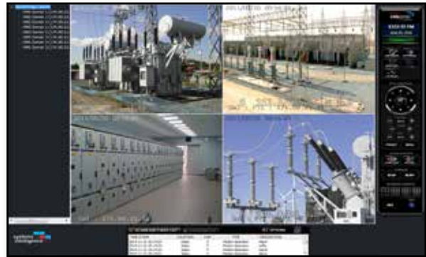
VMS2000 Client Main Screen.
